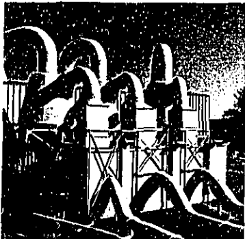
After acoustical treatment of these dust collectors, nearby residents are no longer bothered by noise.
