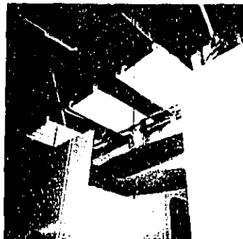
Ceiling baffles incorporate Fiberglas material and perforated metal.
