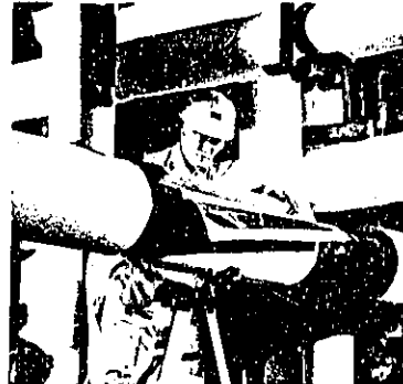
Pipe coverings muffle noisy piping systems. They are also effective unit sound absorbers.
