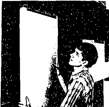
Fibreglass baffles reduce excessive reverberant noise in large, open building areas.
