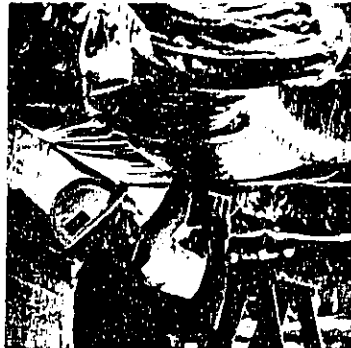
Duct wraps and liners reduce transmission of noise through heating and ventilating systems.
